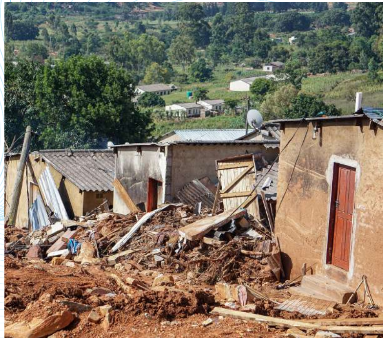
Evidence Chenjerai, GpJ Zimbabwe : Cyclone Idai brought mudslides, boulders and rainfall to the Ngangu area of Chimanimani in March 2019.
